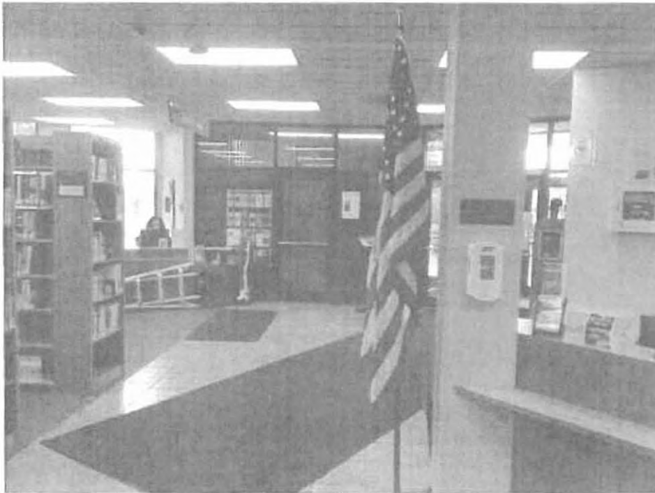
Photograph 7 - Space and Ceiling below Beam B5 at Column
