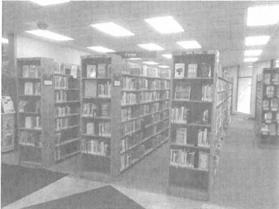
Photograph 8 - Space and Ceiling below Beam B6
