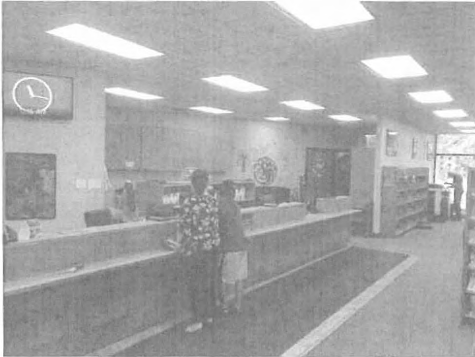
Photograph 6 - Space and Ceiling below Beam B4
