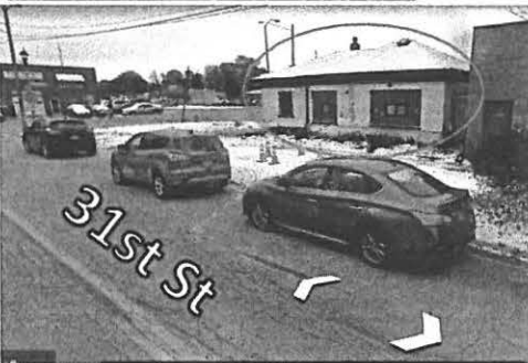
Street View - North Elevation:
